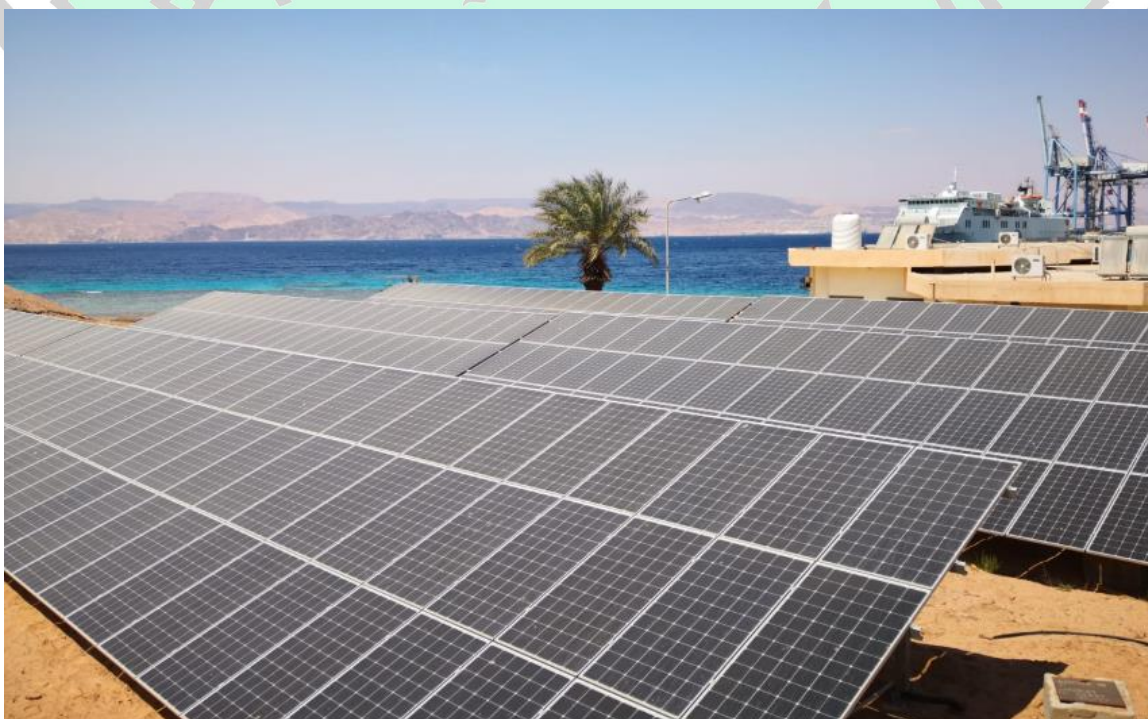
Figure 10 Ground-mounted solar PV system installed at the Marine Science Station.
