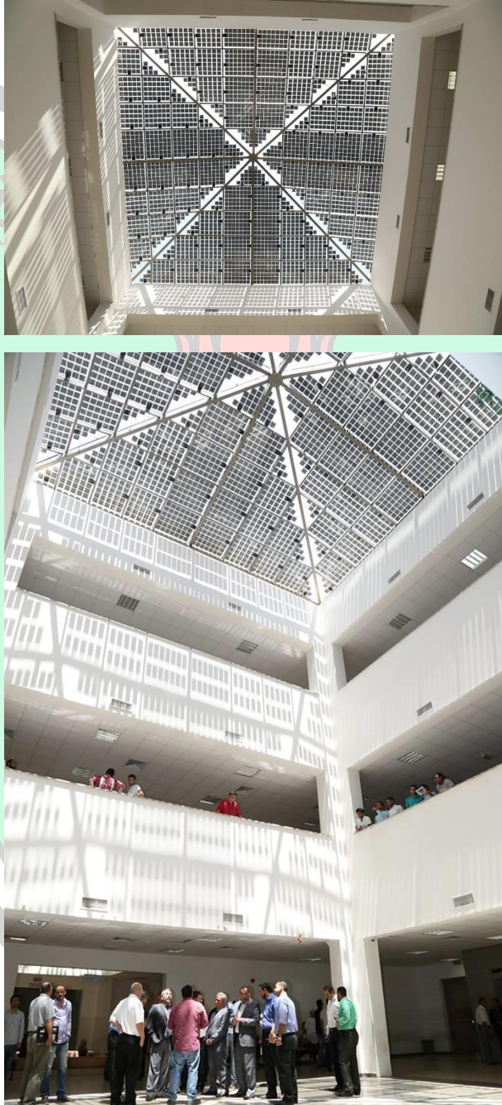
Figure 9 Solar BIPV installed in Aqaba branch.
